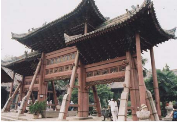
a. Entrance Gate
